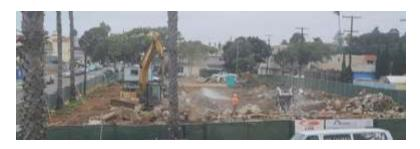
**Oceanside Navigation Center –** The fire sprinkler and fire alarm contracts are being executed this week. The contractor continued coordinating the existing storm drain line with the new lateral sewer work, building new walls, and completing electrical rough-in. The contractor will begin relocating the electrical panel in the coming week.
