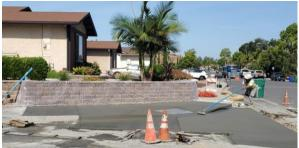
**Brooks Street Swim Center Renovations** – The contractor completed installation of the new rope anchors and will soon receive Building Department inspection of rebar for the light niches and cantilever deck. Construction continues this week, including performing wading pool work, installing new drain lines, and excavating slot drains
