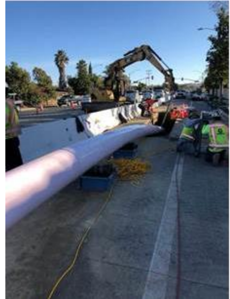
Recycled water main pulled through casing
