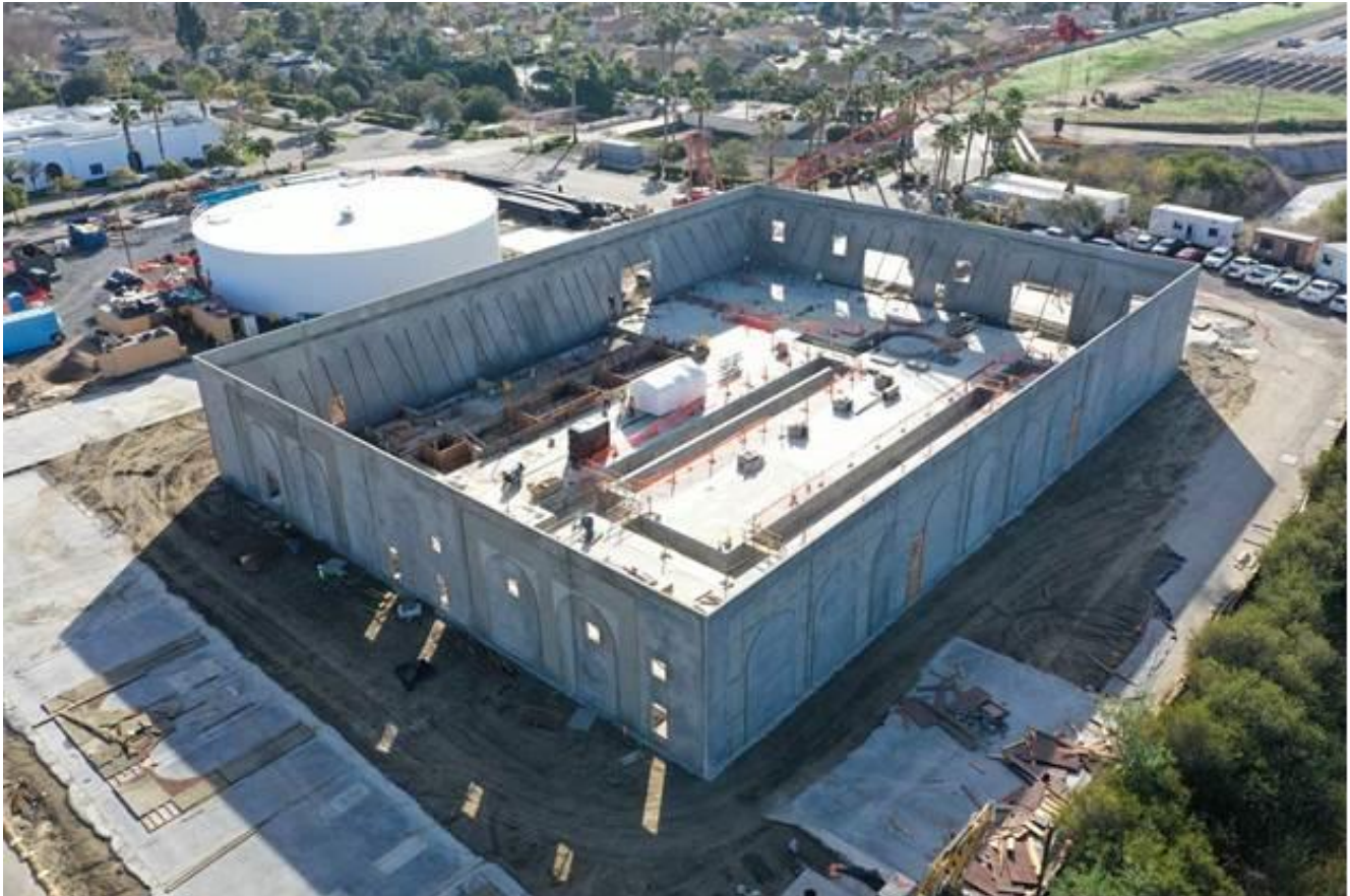
AWPF wall construction with temporary bracing
