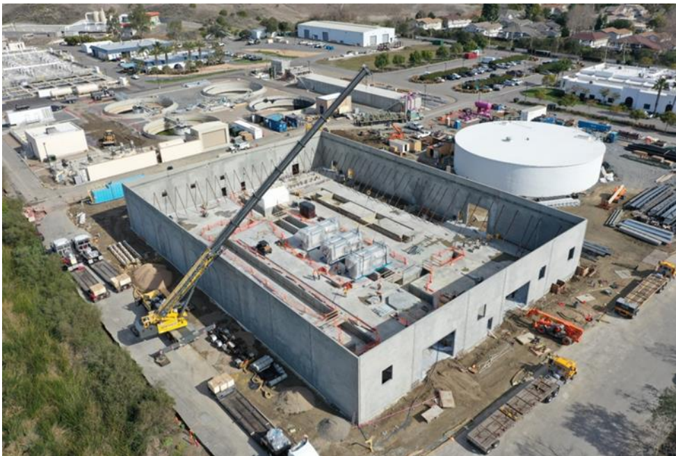
Photo - AWPF RO Skid Hoisting
