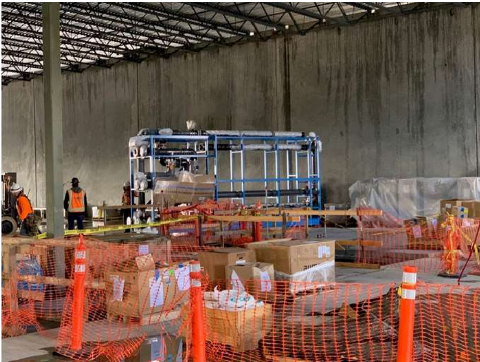
Photo – UF Skid Construction
