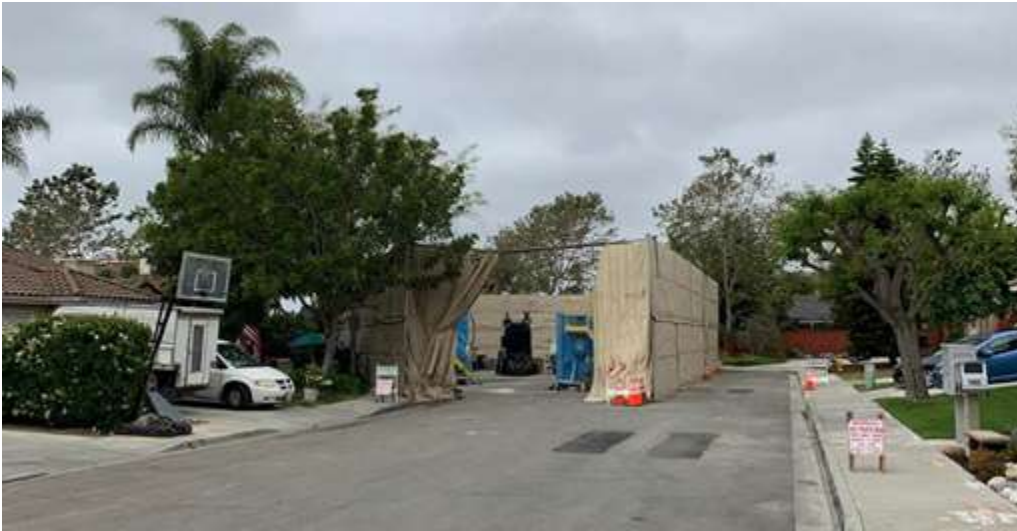
IW-3 on Alizpaz, Drill Rig Demobilized
