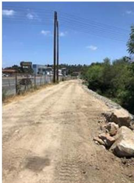
Figure 2 - After the Repairs (June, 2020)
