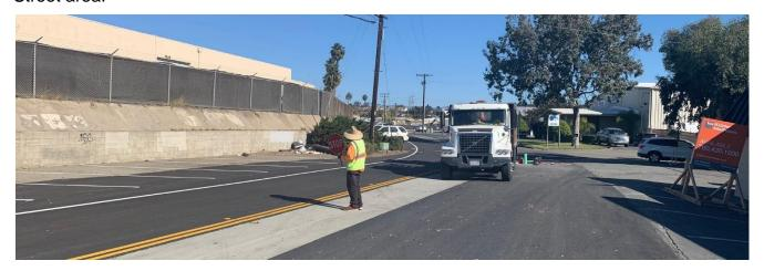
San Ramon/Rancho Del Oro Traffic Signal – Two existing street lights were removed. All traffic signal poles were installed. All wiring, equipment and street signs were attached to the poles. Mill and overlay of Rancho Del Oro Drive will be done on this week as well as the layout of the stripping and advanced traffic signal loops. Signal activation may occur as soon as next week.
