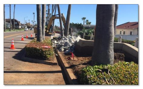
in one seating area at a time and involves removing the concrete stem walls, leveling the soil in the adjacent planters to match the elevation of the sidewalk and removing/replacing plant material which is consistent with the existing design. In addition, all benches will be replaced. The work will not significantly change the overall feel of the area but should aid OPD with their patrolling efforts as well as ease the maintenance issues.
