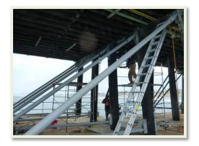
**Municipal Pier Brace/Bracket Replacement Project**Ballard Marine is moving along on the replacement of steel pipe braces/brackets on several sections of the pier. The project is anticipated to be completed by late September.
